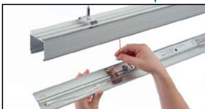
Secure electrical unit to trunking with security cable
